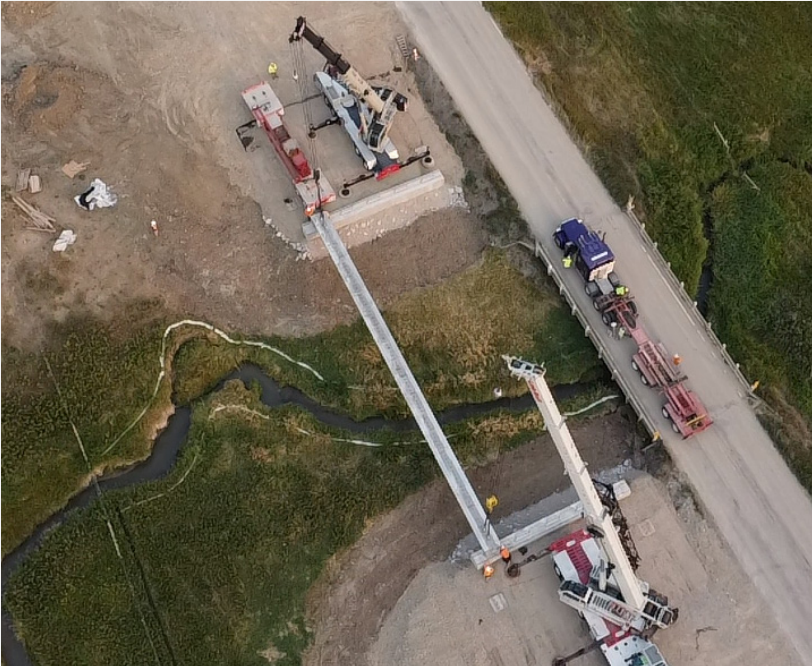
Setting of the first girder with a two crane pick.
