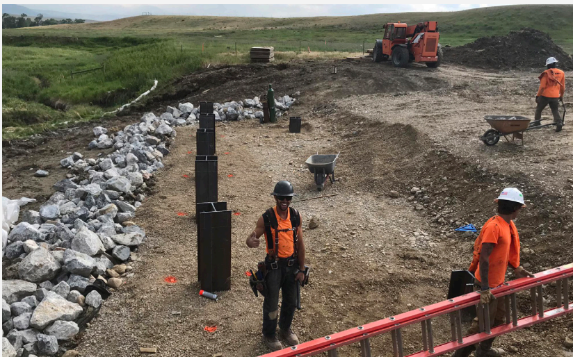
Driving piles on the west side of the bridge.
