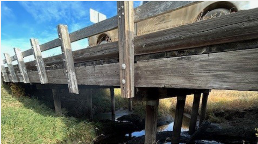
Wheatland County Bridge prior to construction.
