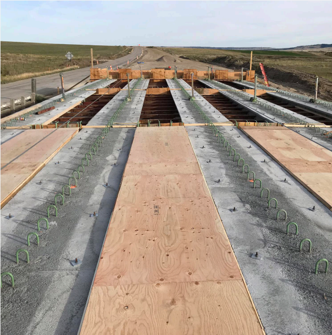
Soffit forms for the cast in place deck.
