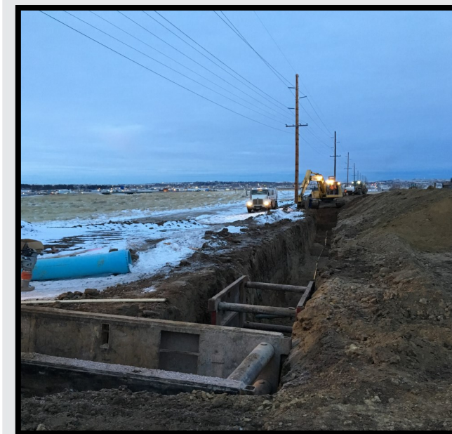
18" water main trench along Highway 51 in Gillette, Wyoming.
