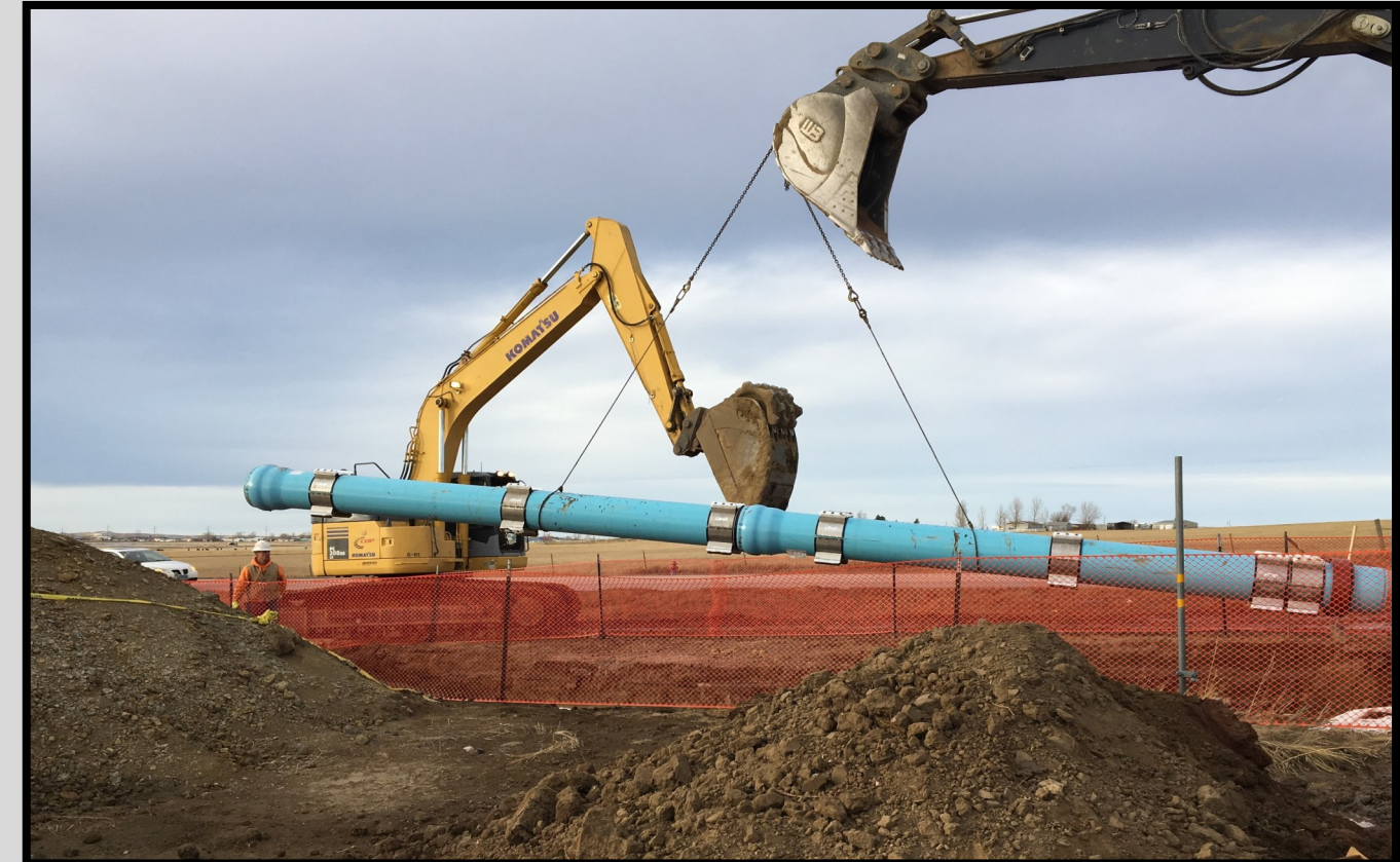
Crew installing 18" restrained pipe with chocks for 30" bore.
