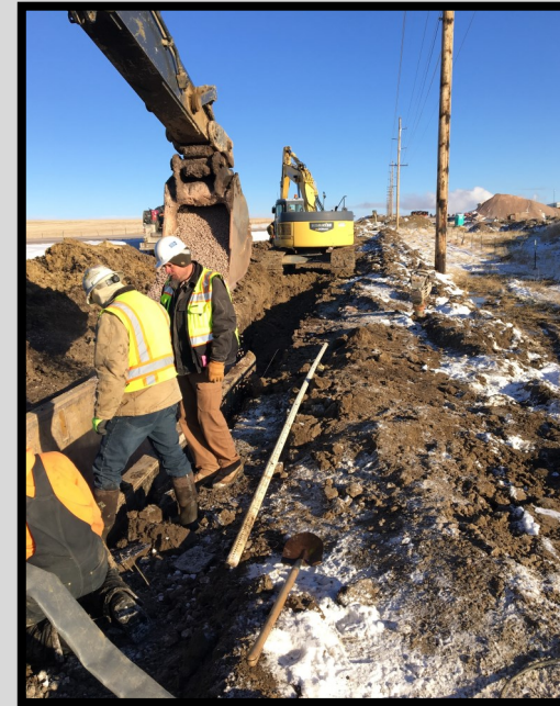
Crew installing 18" water main near Highway 51.
