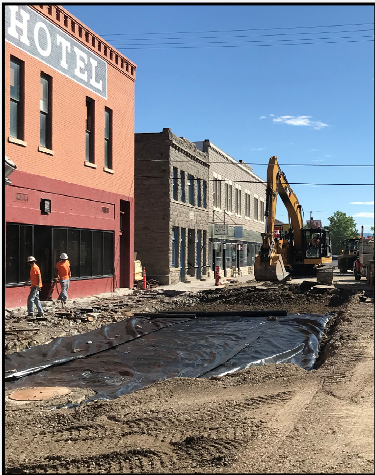
Street excavation on Callender Street.
