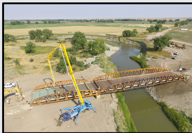
Pouring the bridge deck on the new 2 span steel truss bridge.
