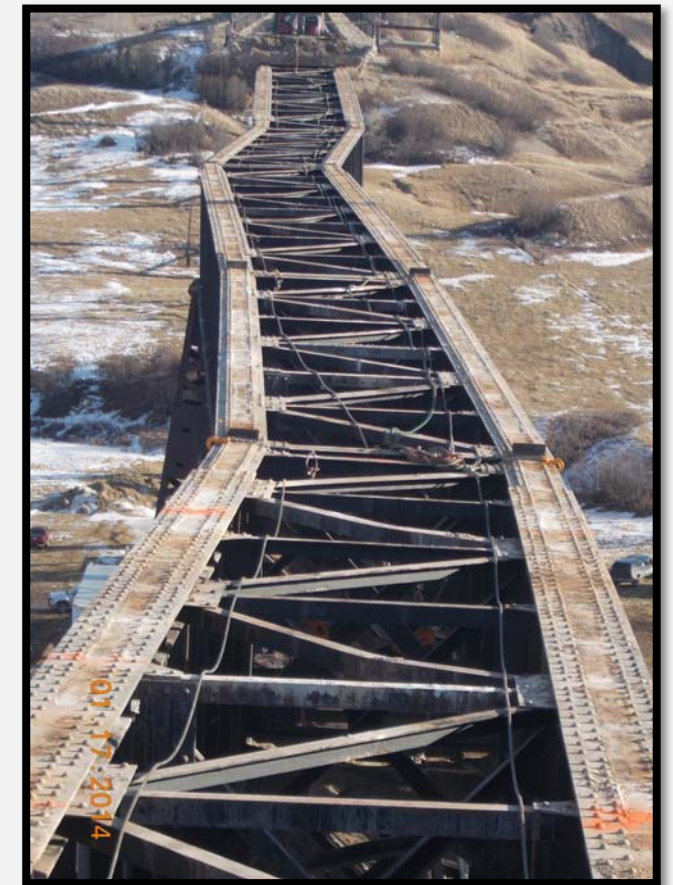
Tops of Girder Spans, Before Demolition, Looking South.
