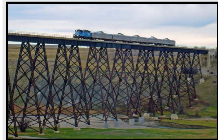
Completed Judith River Trestle Project
