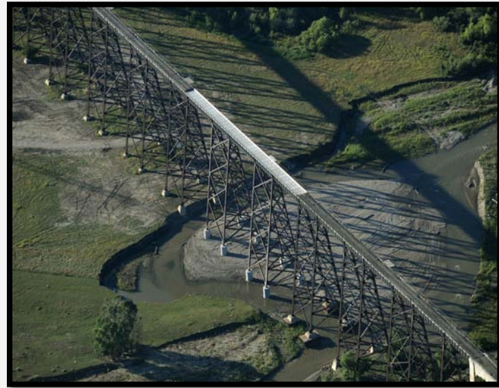
Aerial view of completed project.
