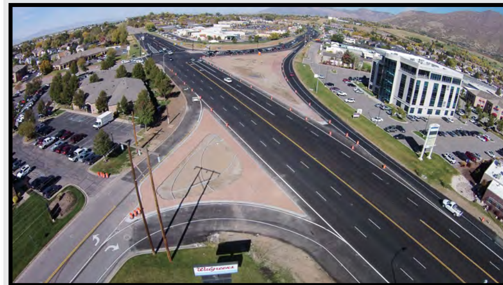
Aerial view of completed project.
