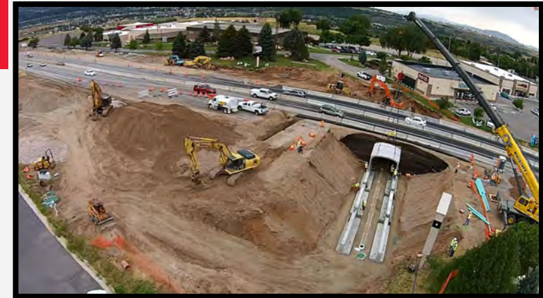
Installation of Pedestrian Tunnel.
