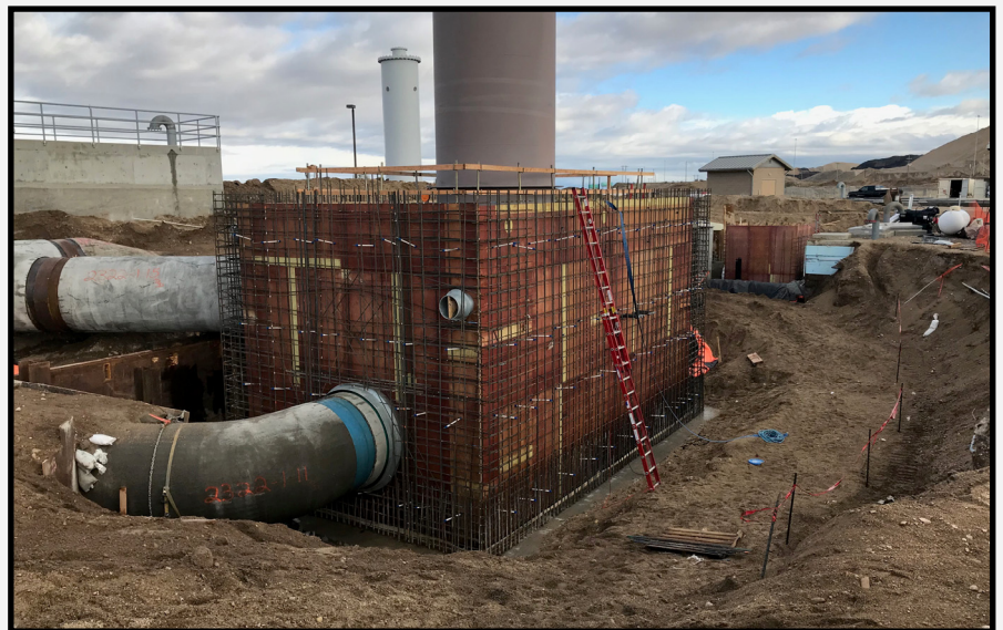
Point of the Mountain flow control structure.
