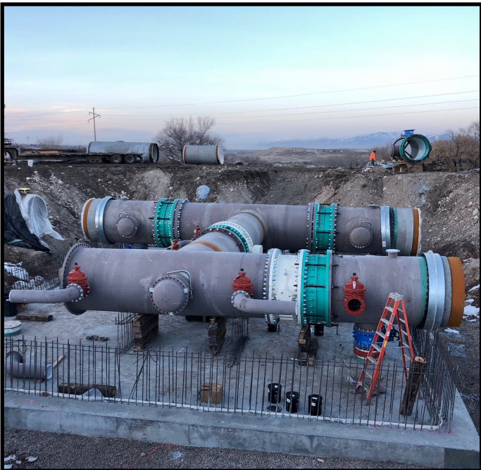
Jordan Narrows Pipeline Interconnection vault in different phases.
