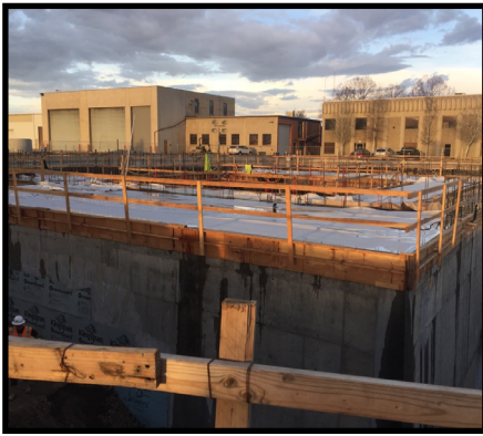
Installation of the new 48-inch sewer, 25-feet deep.
