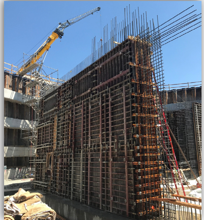
Concrete forms constructed to pour the walls of the structure.
