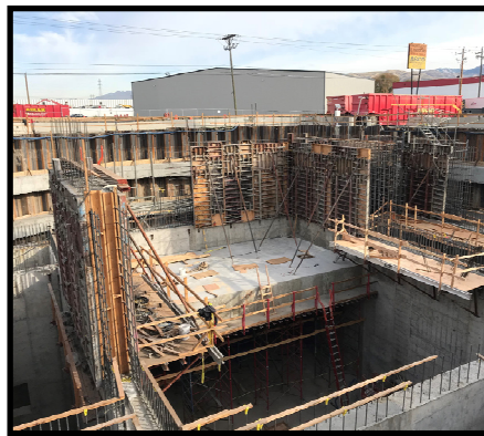
Concrete forms constructed to pour the walls of the structure.
