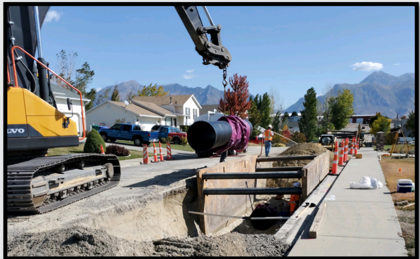
Setting 30-inch ductile iron pipe down a residential street.
