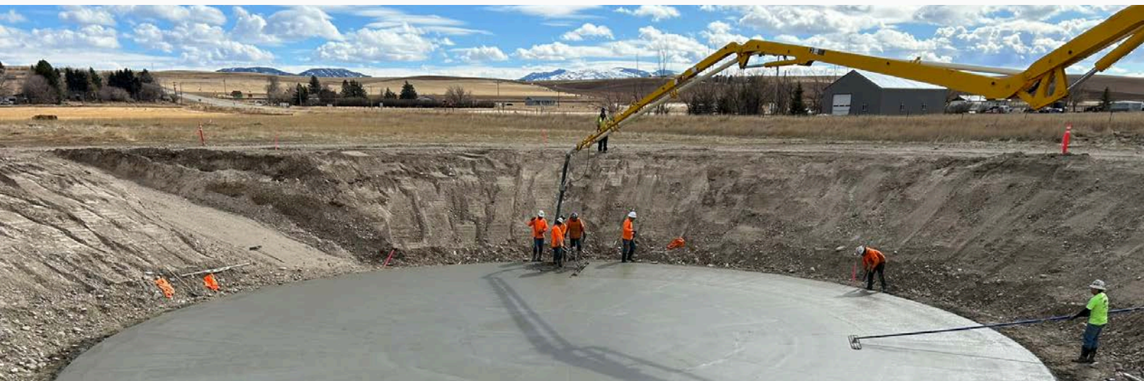
Tank foundation on the Townsend Water Improvements Project
