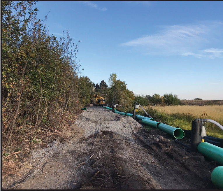
Dewatering wells through the wetlands.
