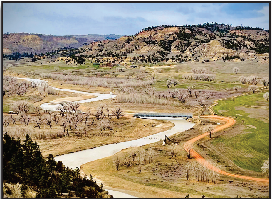
Overview of the Moorhead Bridge from a local trail.
