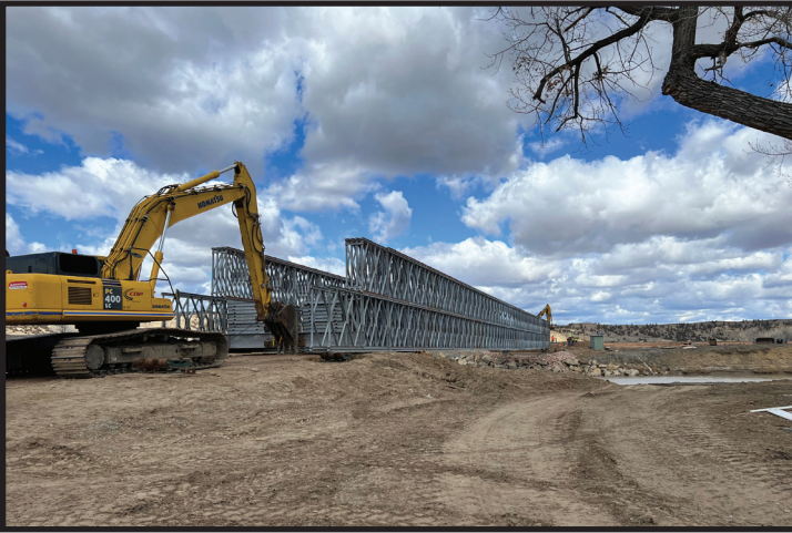
Bridge being pushed out across the Powder River.
