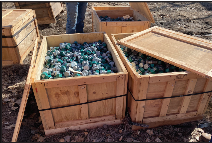
Lots of bolts to install.
