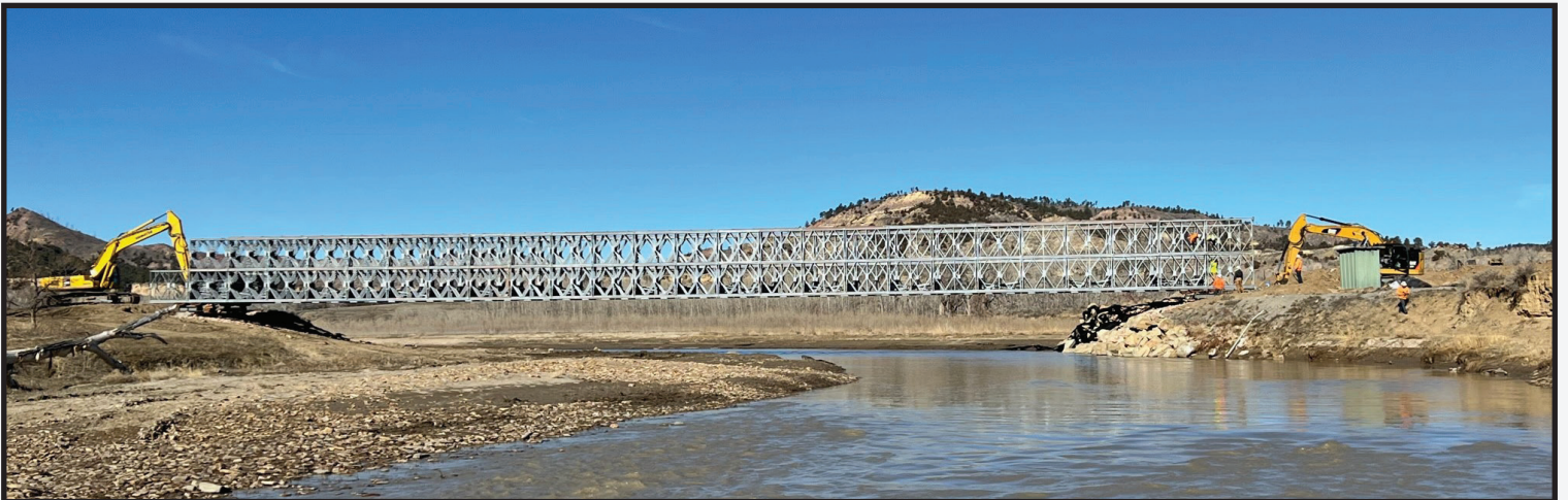
Lowering bridge onto revised abutments.
