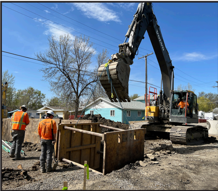
Storm Drain installation near the intersection of South 4th Street and Woodland Avenue.
