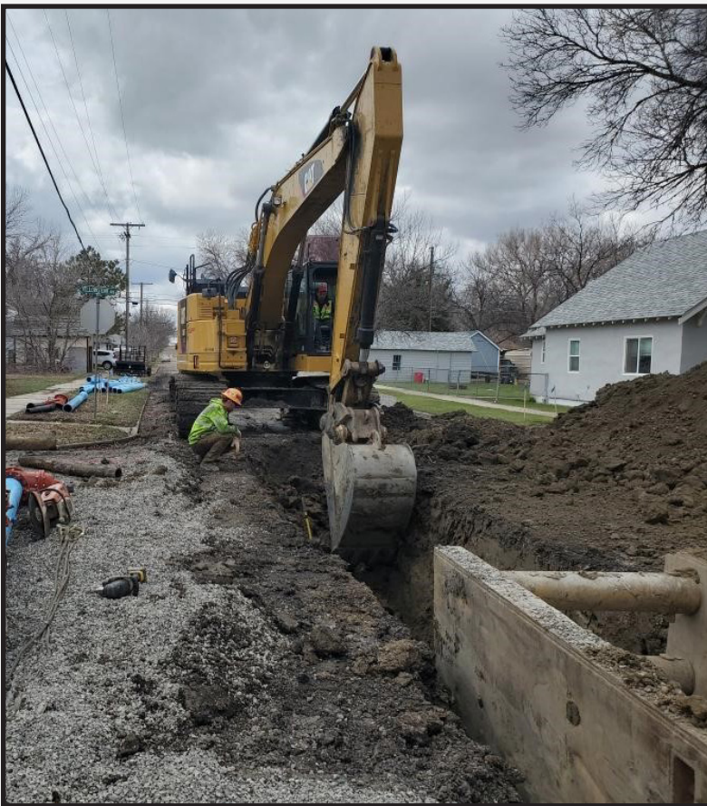
Water mainline installation on South 4th Street.
