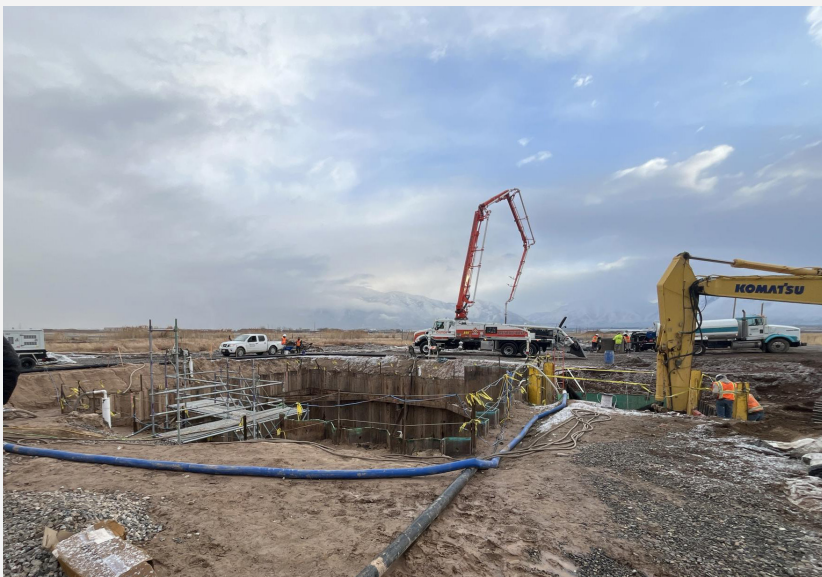
Lift station foundation placement.
