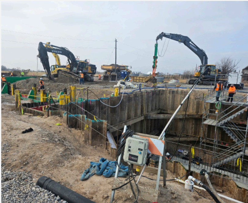
24" deep sewer installation.
