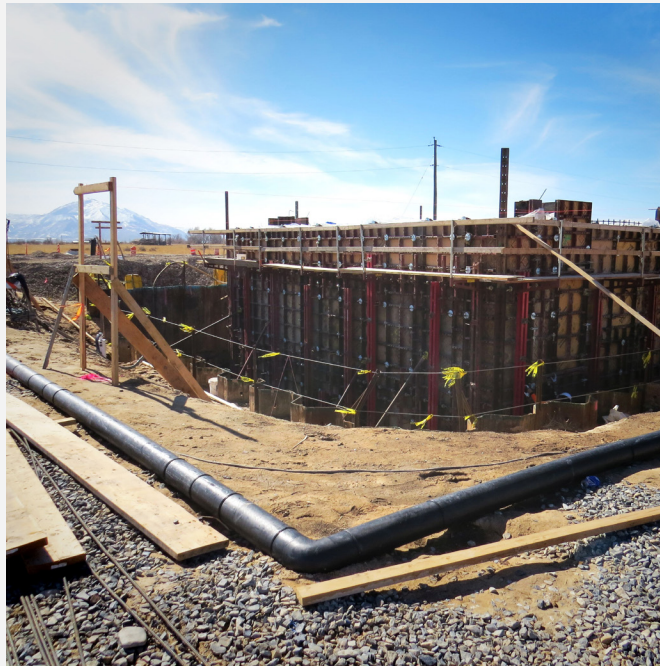
Lift station exterior wall forms.
