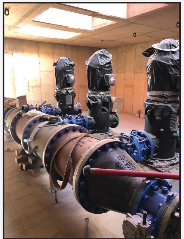
Installing 3 each vertical turbine pumps and mechanical piping inside the pump station.
