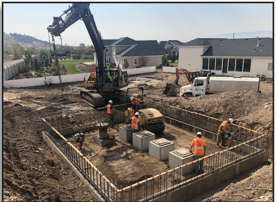
Backfilling pump station in preparation for a slab on grade pour.
