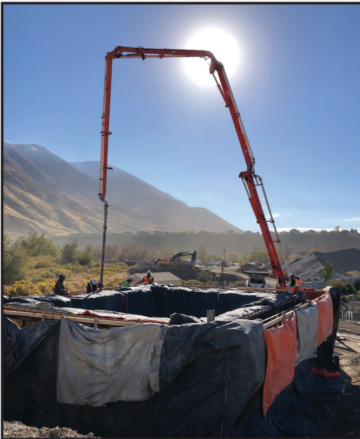
Pouring the pump station walls.
