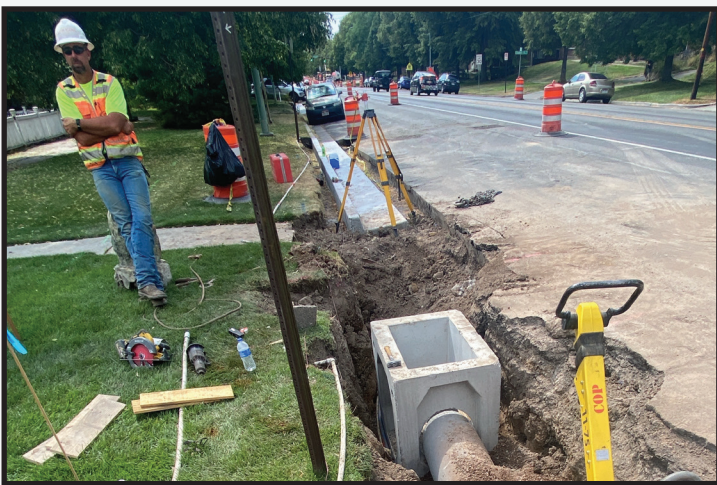
Storm drain installation.
