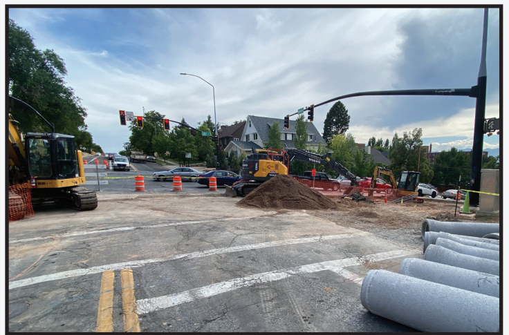
University Ave & 100 South intersection storm drain reconstruction.
