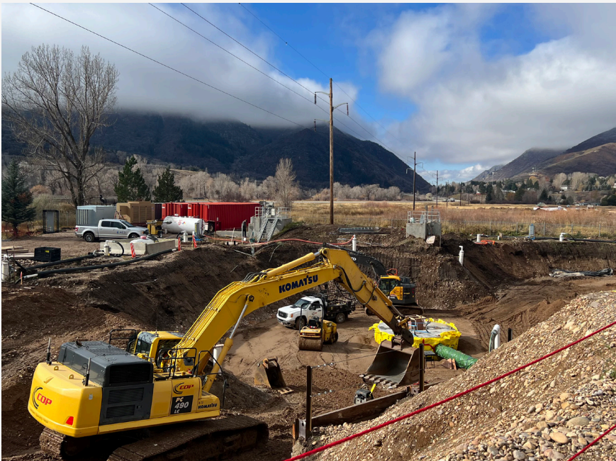
Finishing grade for clarifiers.
