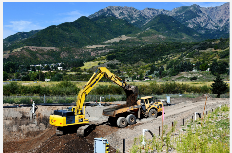
Excavation for clarifiers.
