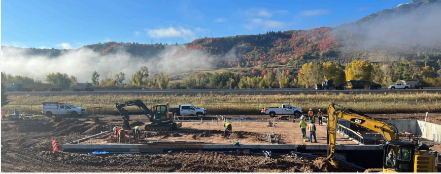
Finishing grade for the plant operations building.
