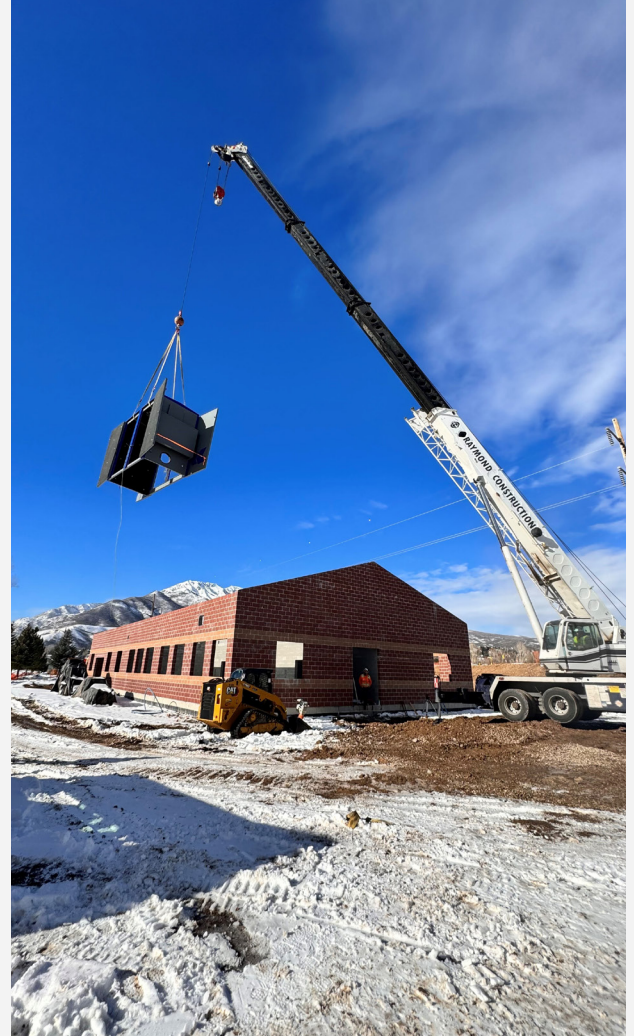
Blowers for the plant operations building being placed.
