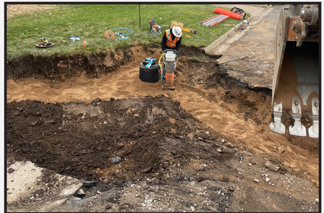
COP Crew compacting backfill after a new 1" water service was installed.
