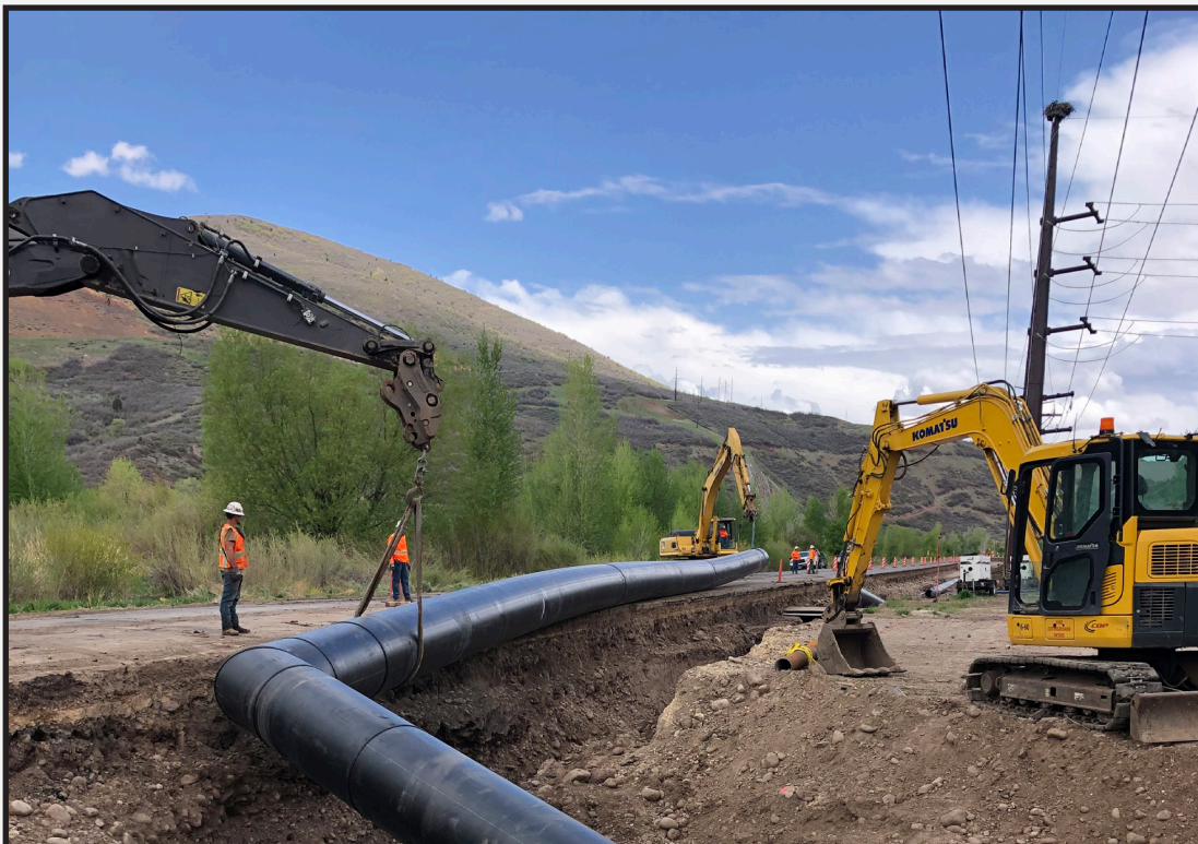
Installing our prefabricated 42" HDPE tie-in section on the projects south end.
