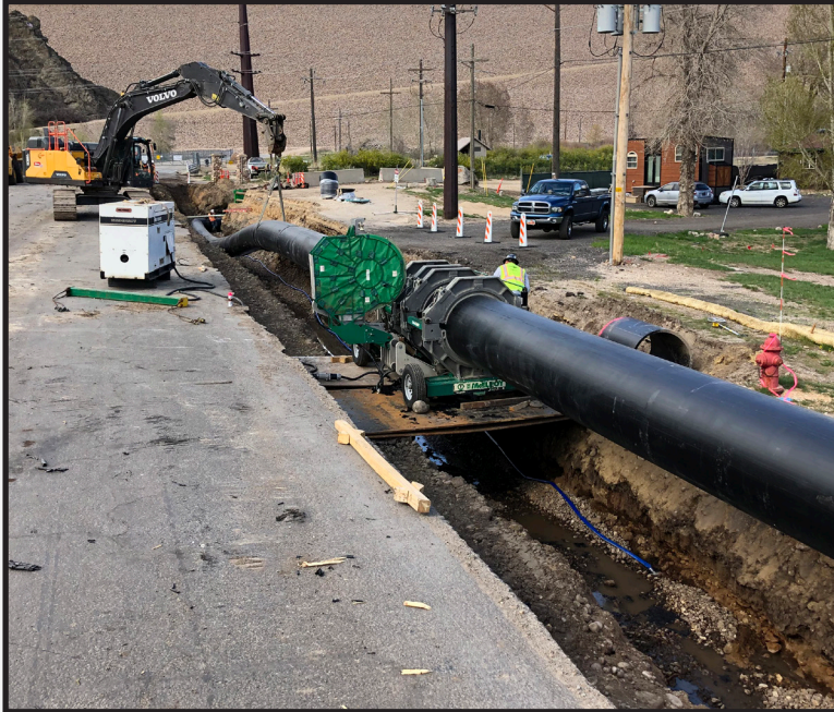
Fusing 42" HDPE after installing our prefabricated tie-in section that had to be stabbed under existing utilities on the projects north end.
