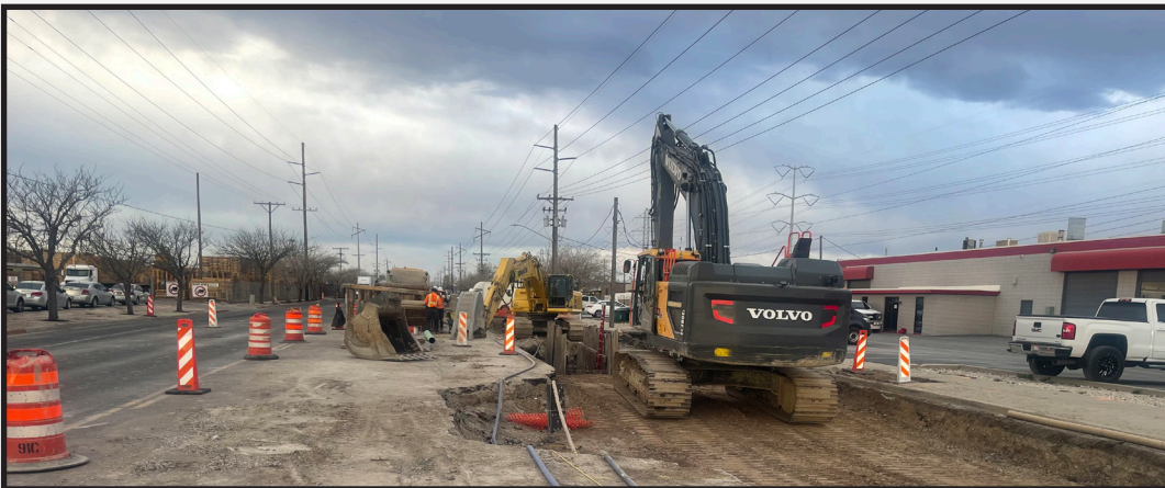
Excavation for manhole number three
