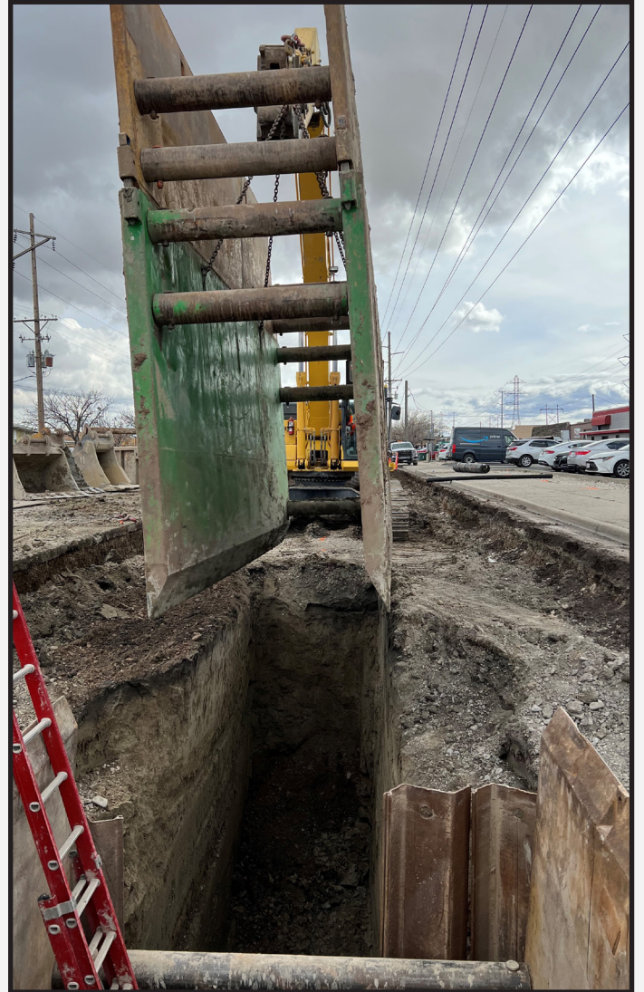
Installation of mainline double stacker trench box
