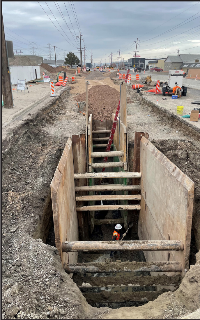
Excavation for manhole number three
