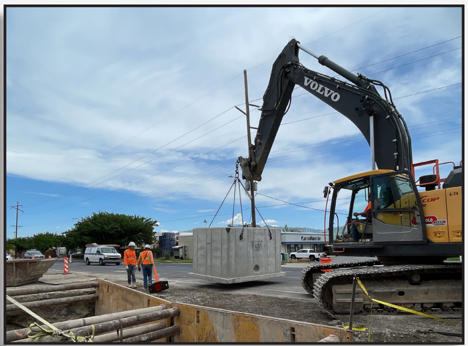
Installation of Force Main Pig Retrieval Vault
