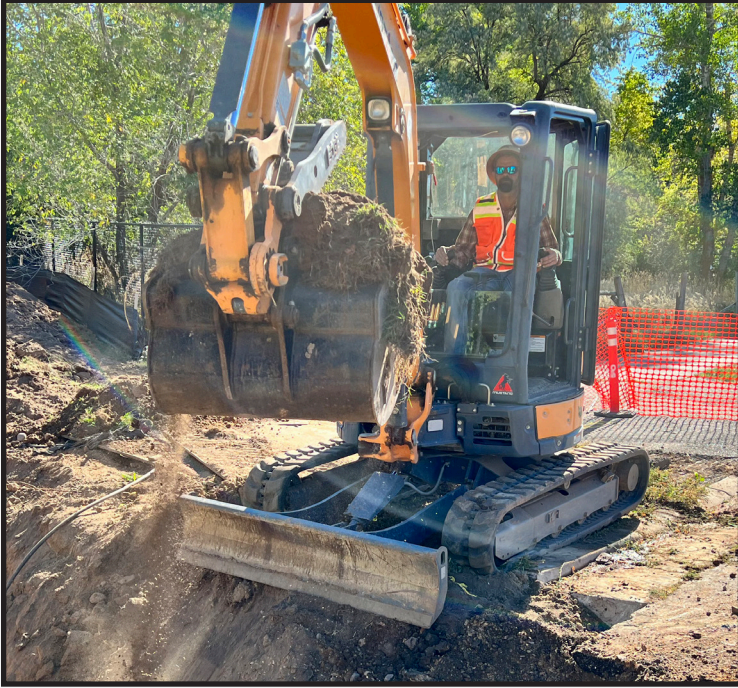
COP Crew excavation for tie-in of the 20" discharge waterline.
