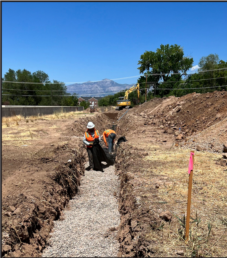
Crew backfill of newly installed 20" suction waterline.
