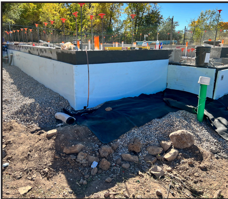
Pump station building foundation completed.
