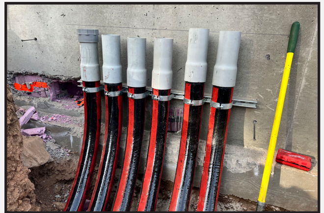
Turner Electric installed conduit risers at newly constructed pump station building.
