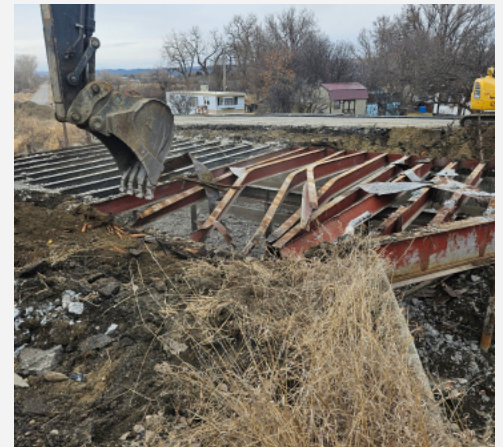
Removal of 20 steel girders originally placed in 1925
