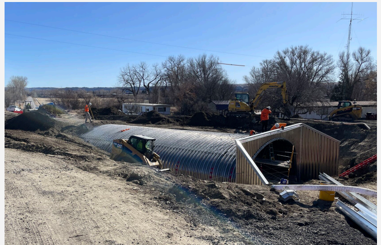
Installing the headwall and wingwall anchor rods and backfilling the structure
