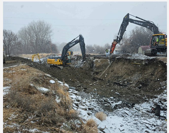
Demo of the abutments and excavation
