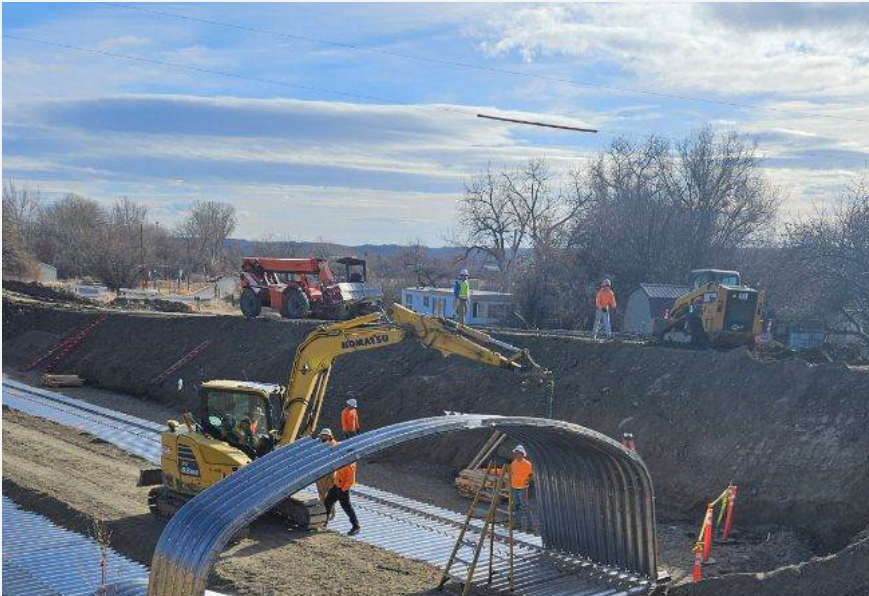
Installing the haunch and crown pieces of the structure
