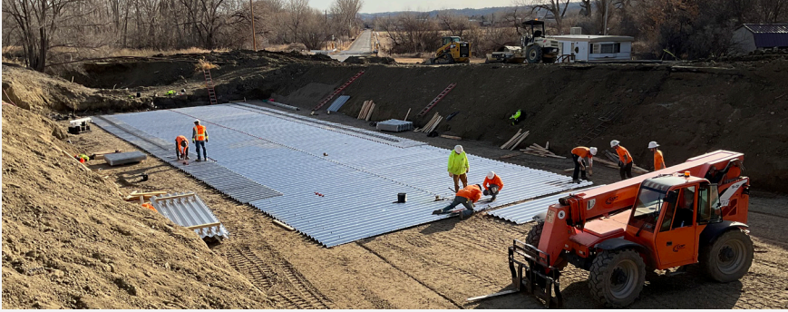
Installing the invert panels for the base of the structure
