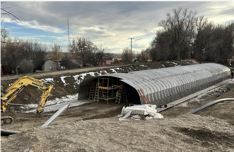
Installing the haunch and crown pieces of the structure
