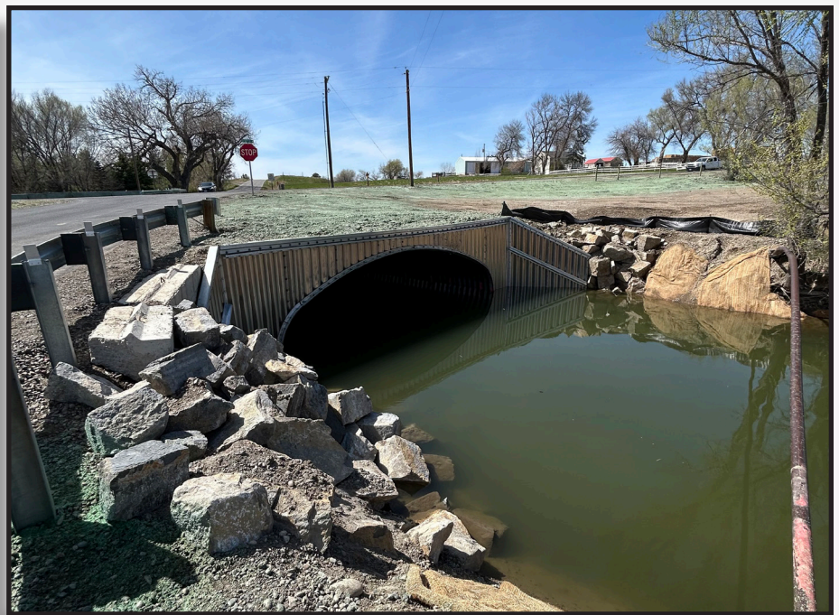
Finished new culvert
