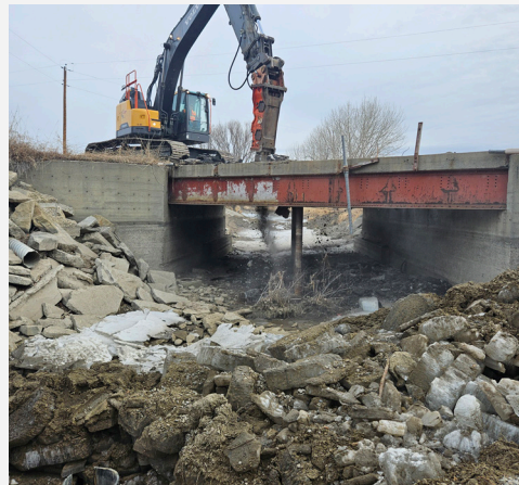
Demo of asphalt & concrete deck
