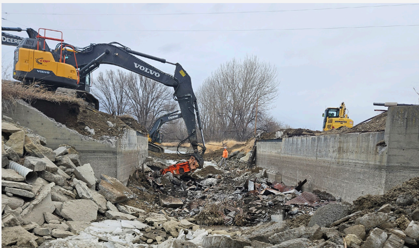
Demo of the abutments and excavation
