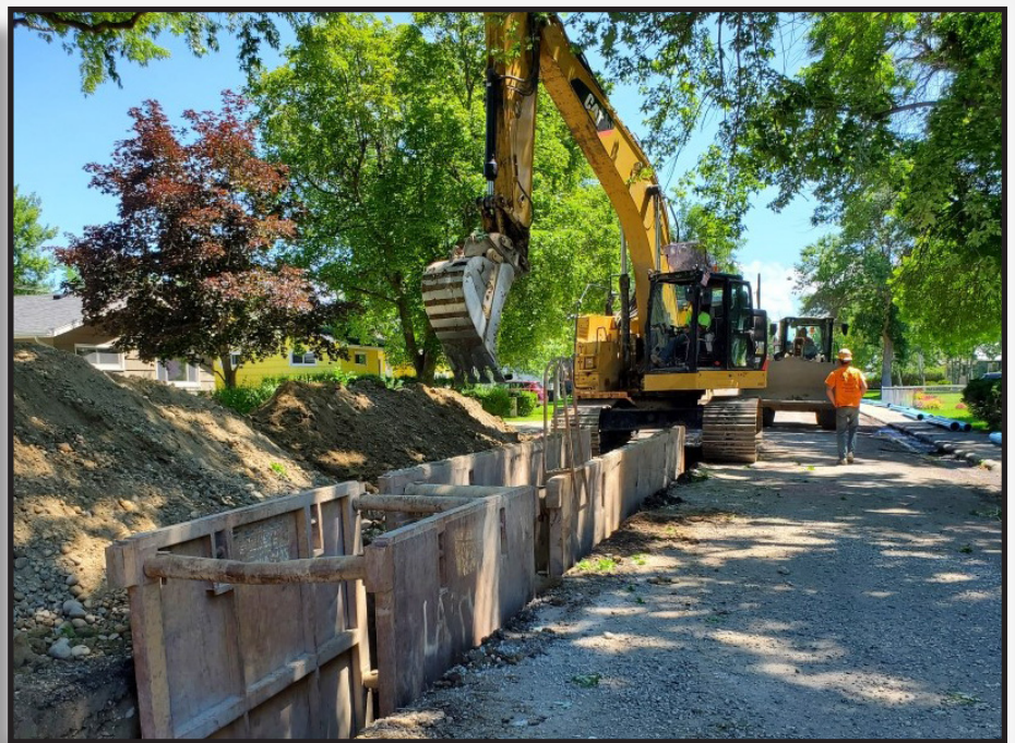
8" Water Main Replacement at the 1000 Block of Avenue F.
