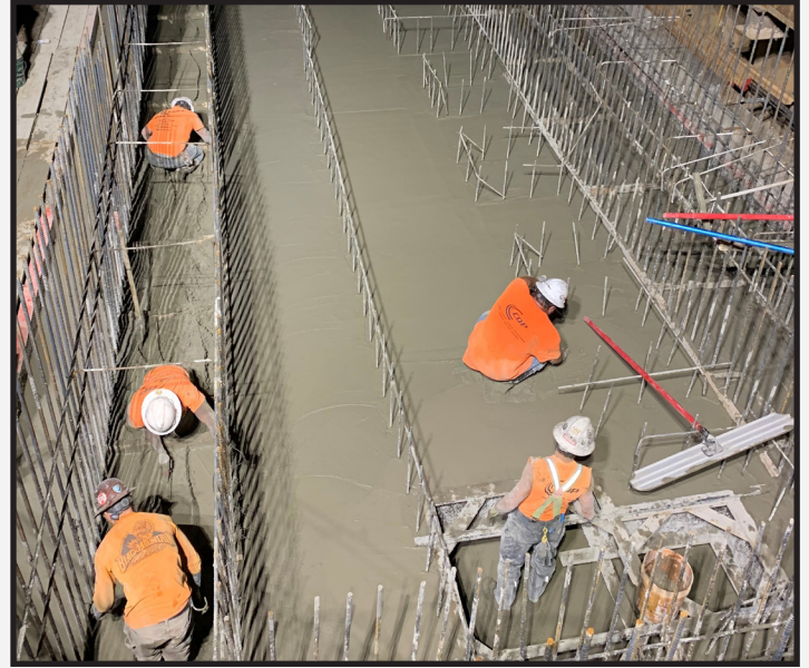
Finishing wet well base slab concrete.
