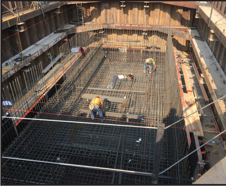
Tying wet well base slab rebar.
