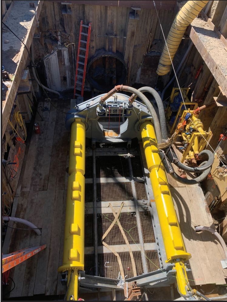
Micro-tunnel jacking frame.
