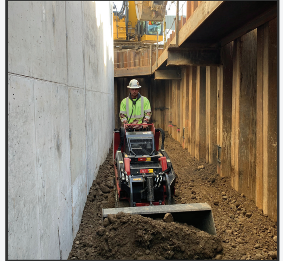
Backfilling wet well.
