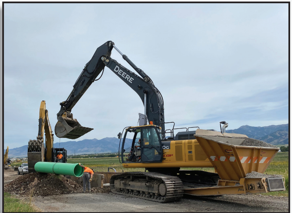
Installation of pipe to lift station.
