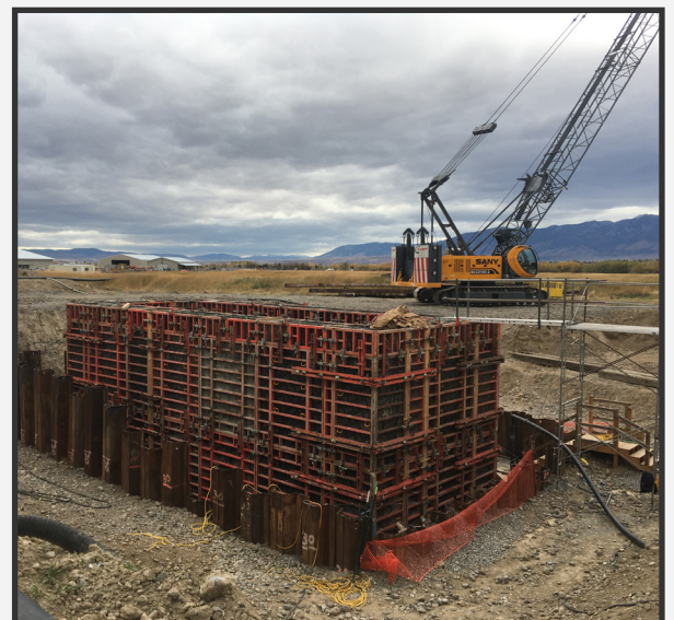
Lift station wall forms.
