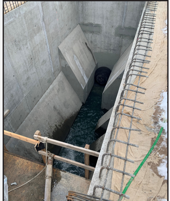
Filling the wet well for the water test.
