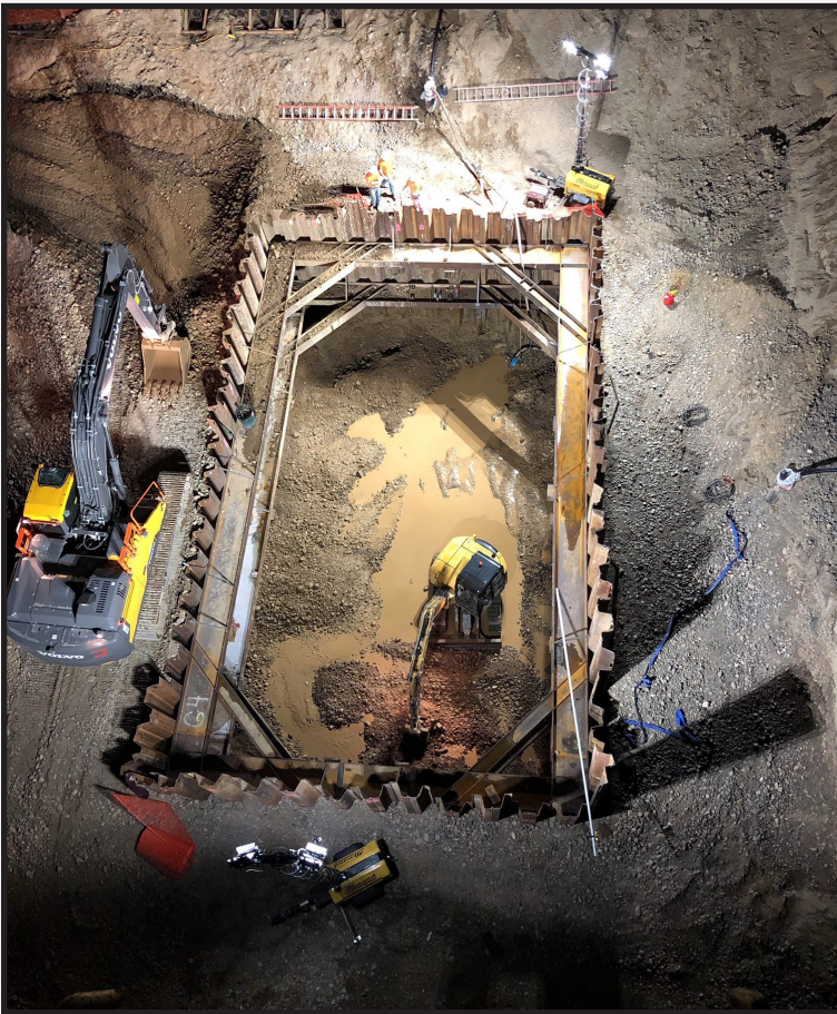
Wet well excavation.
