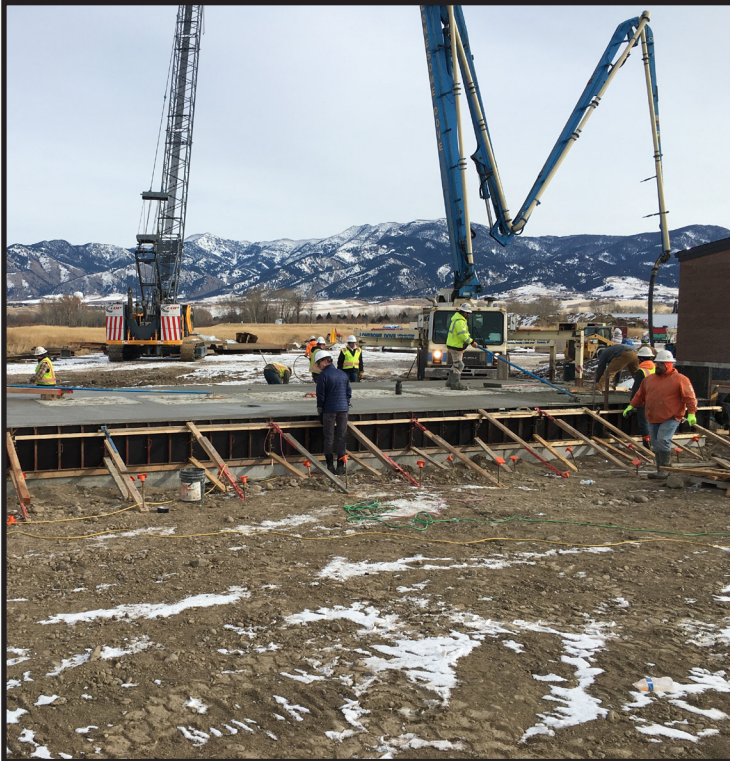
Pouring the lid of the wet well.
