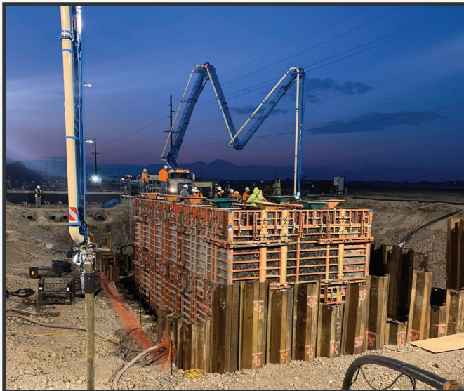
Pouring the wet well walls, 410 cubic yards of concrete.
