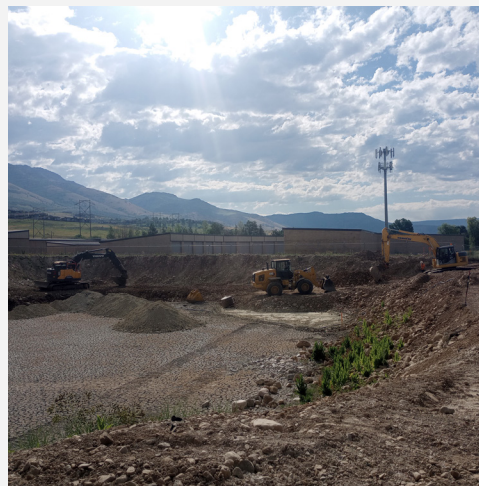
Grading and placement of Bentonite Pond Liner
