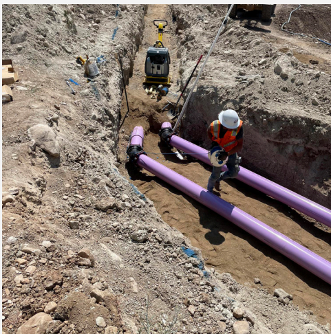
Installation of Reuse Project pipelines
