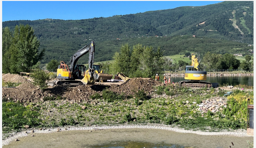
Initial earthwork for sewer lines and access road.
