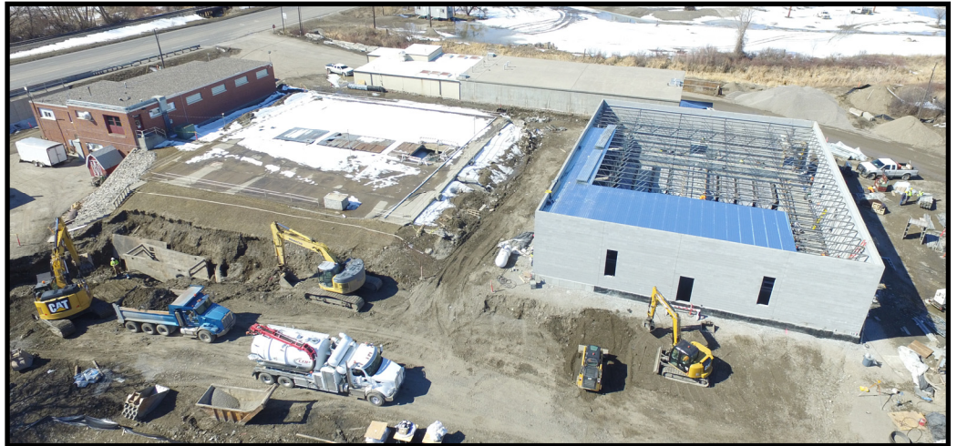
The Laurel Water Treatment Plant in different phases of construction.
