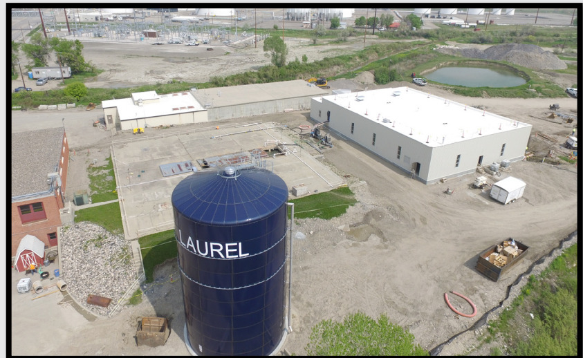
Aerial view of the Laurel water treatment plant.
