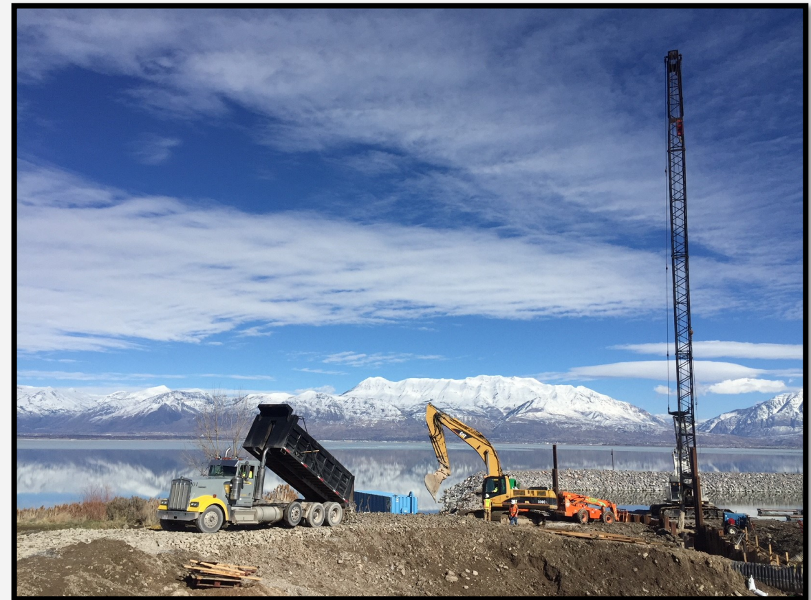
Establishing the road down to the intake structure.
