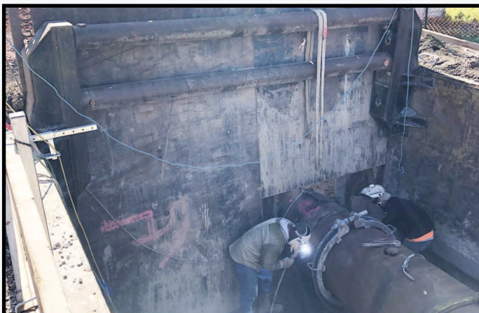
Installing 212 linear feet of 30-inch diameter with our pneumatic hammer.
