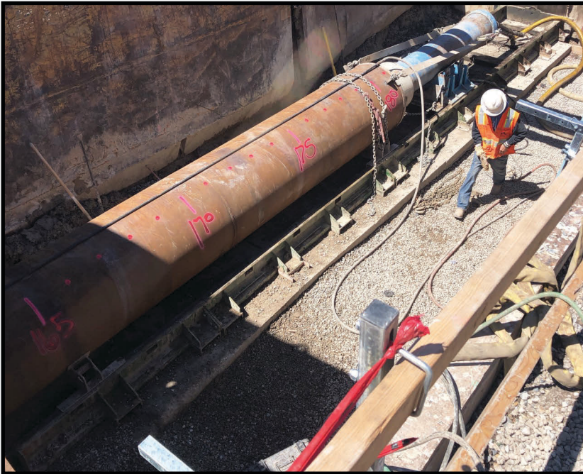
Installing 212 linear feet of 30-inch diameter with our pneumatic hammer.
