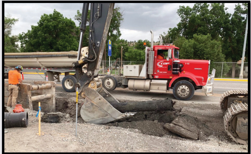
Removal of existing watermain.
