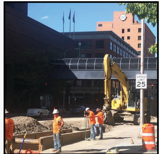
Pouring flow fill in MDT right of way.
