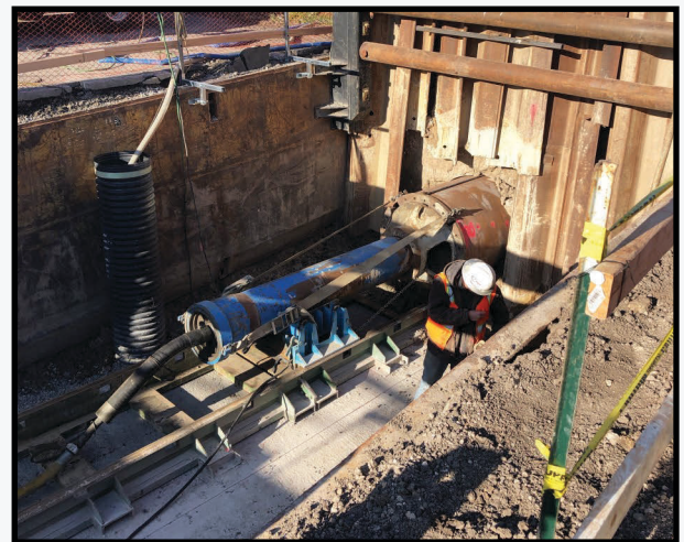
Installing 212 linear feet of 30-inch diameter with our pneumatic hammer.
