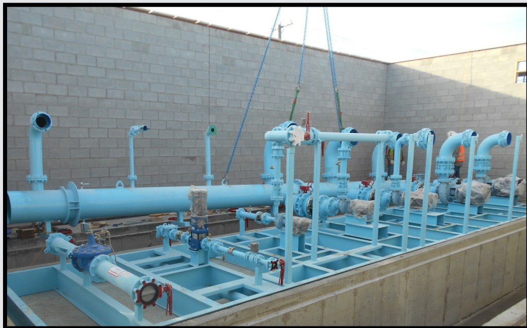
Installing the new skid mounted pump station in the building.
