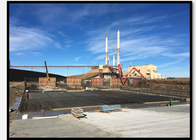
One of many base slab pours.
