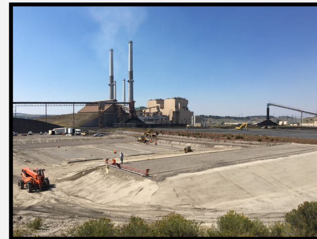
Preparing for the first mud slab pour.
