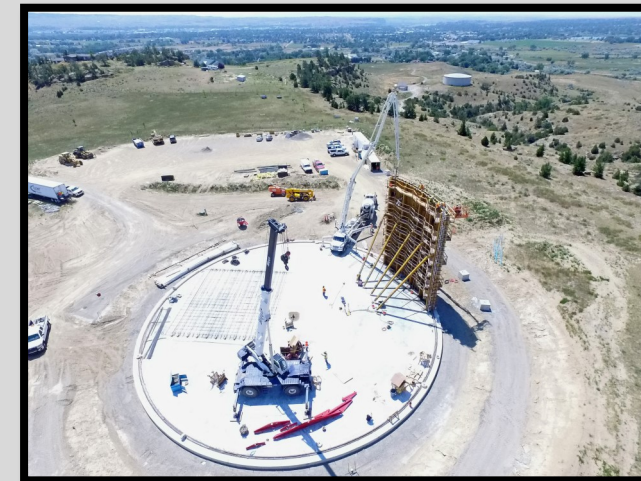
3. Drone shot of first wall pour.
